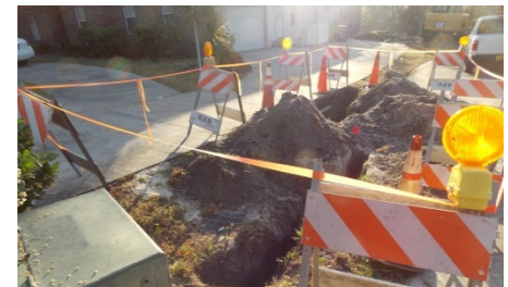
Removed and replaced drainage system on North Ridge Lane..
