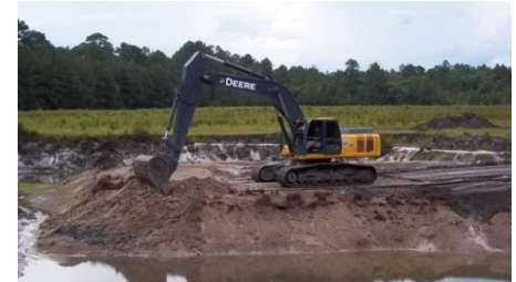
Completed excavation and sloping at Connor Pit.
